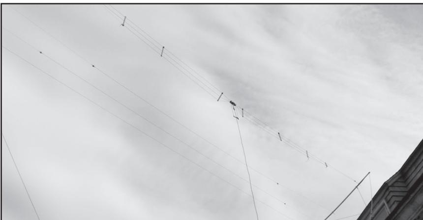
Fig 6—VE7CA portable 2-element wire Yagi installed at Plimoth Plantation in Plymouth, Massachusetts. (Photo courtesy K1HTN.)
